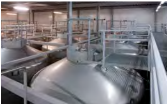
Plant upgrades and maintenance
